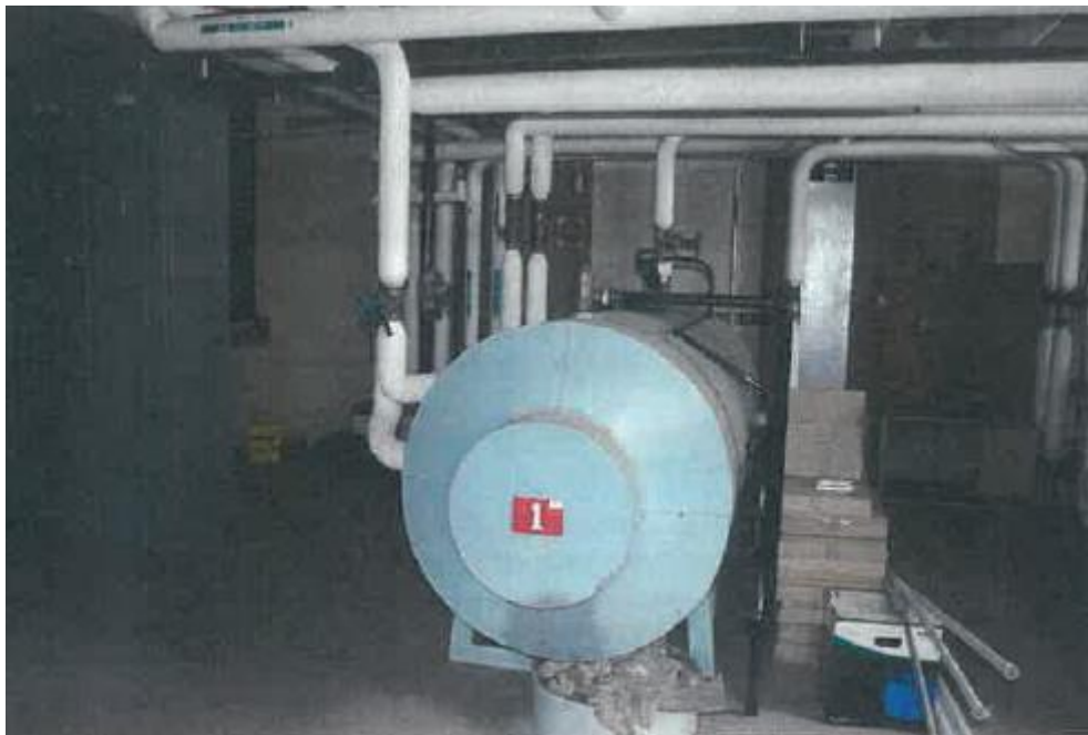
Figure 7 Example of old hot water storage
